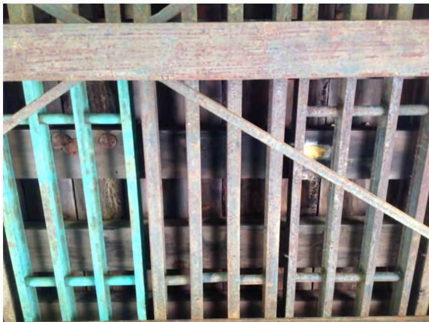
deck from below
