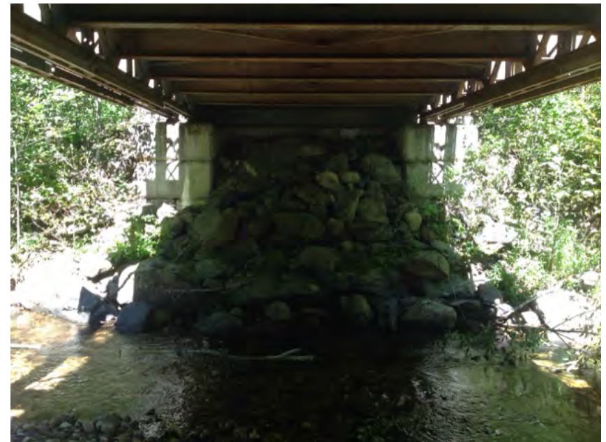
Right Bank Abutment when facing downstream
