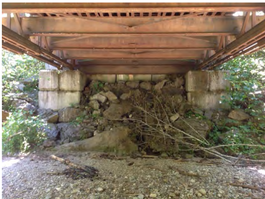
Left Bank Abutment when facing downstream
