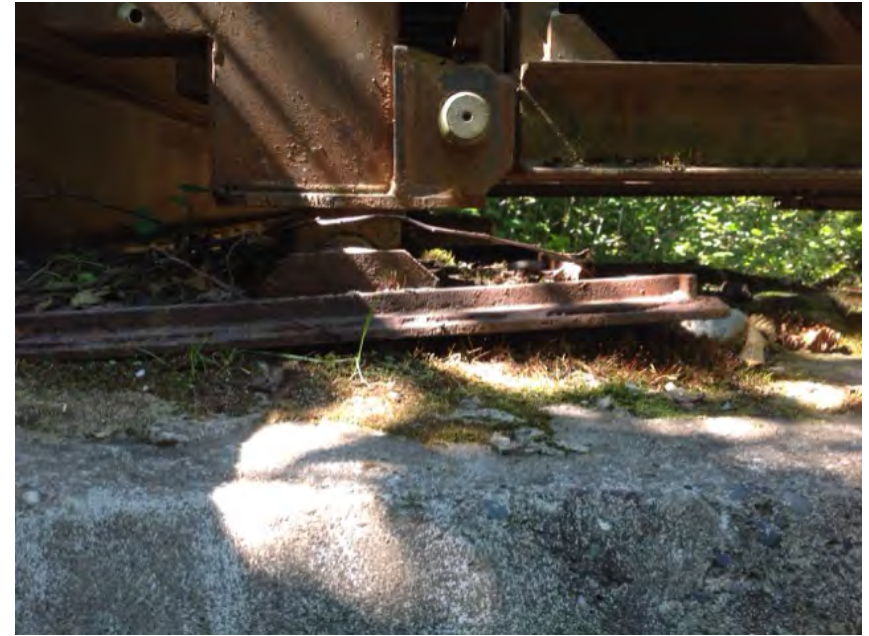
upstream left bank footing
